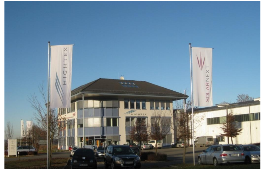
Headquarter at Bernau am Chiemsee
