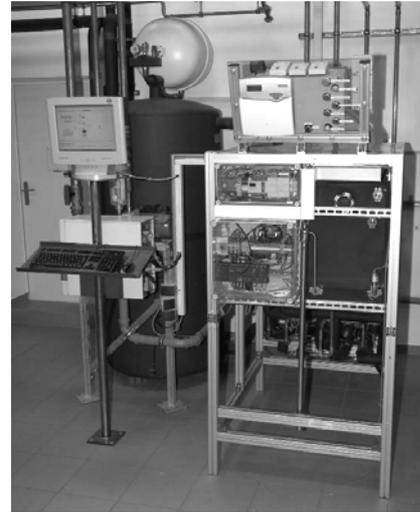
Figure 7 chillii® STC6 with cold storage tank, control and measurement devices
