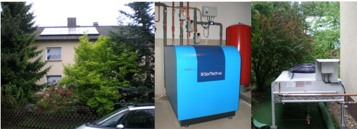
Fig. 5. Flat plate collectors on the roof of the two-family-house as well as the chillii<sup>®</sup> STC8 adsorption chiller and the dry re-cooler (sources: SolarNext).
