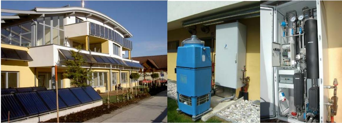
Fig. 6. Flat plate collectors on the facade and the ground as well as absorption chiller chillii® PSC10 at the training center and office building of the company BachlerAustria (sources: SolarNext).
