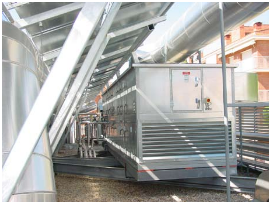
西班牙Mataro实验室中太阳能辅助DEC系统的通风PV正面和太阳能空气收集器 (来源: zafh.net) Ventilated PV facade and solar air collectors of a solar assisted DEC system of a library in Mataró, Spain (source: zafh.net)
