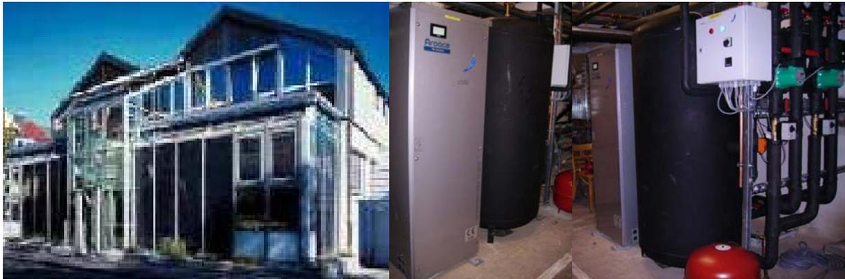
**Figure 5 – Thermal cooling system of a bakery in Germany using a chillii® Cooling Kit WFC18 and waste heat from the exhaust gas of the ovens (sources: SolarNext)**
