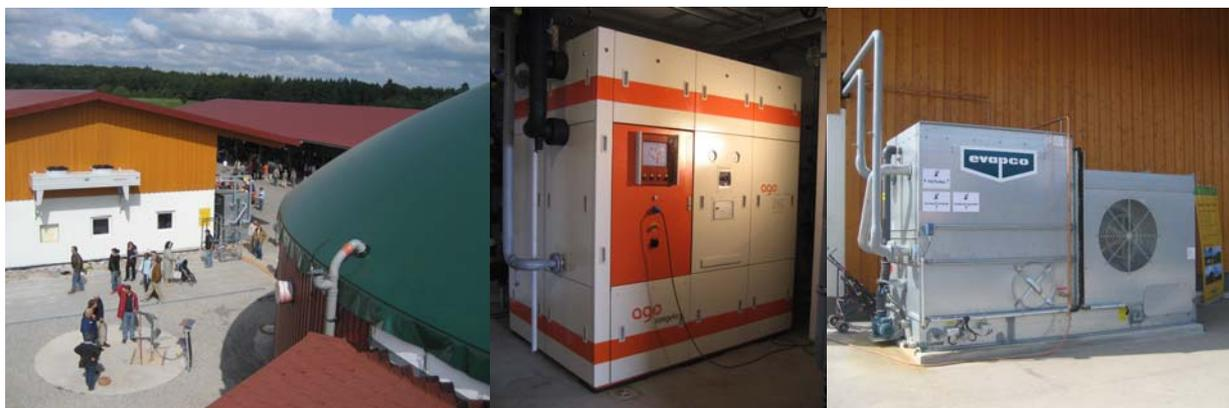
**Figure 6 – Ammonia/water absorption chiller congelo 50 (chillii® ACC50) in combination with a CHP unit for potato cooling in Germany (sources: AGO)**
