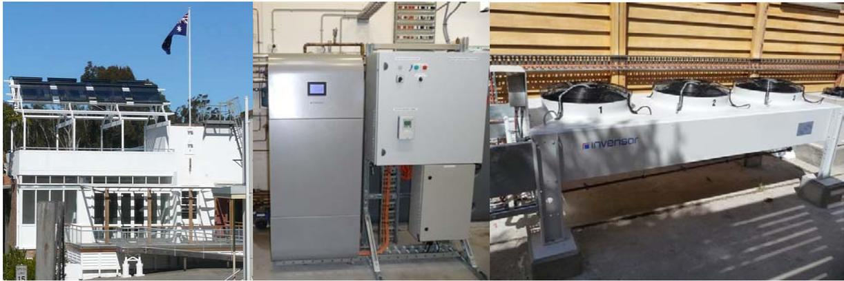
**Figure 7 – Vacuum tube collectors on a special roof construction of a heritage in Australia as well as chillii® Cooling Kit ISC10 consisting of water/zeolith adsorption chiller and dry re-cooler with water spraying (sources: UrbanEnergy)**
