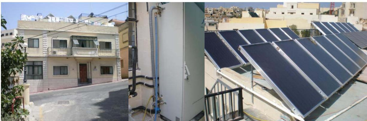
**Figure 4 – chillii® Solar Cooling Kit PSC10 with flat plate collectors on the roof for space cooling of a retirement home in Malta (sources: SolarNext)**
