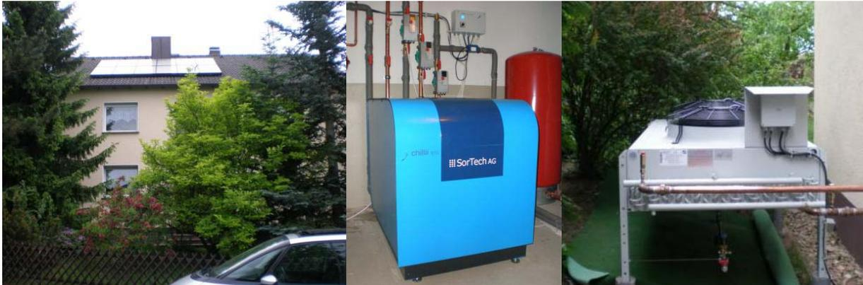
**Figure 3 – Flat plate collectors on the roof of a two-family-house in Germany as well as the adsorption chiller and the dry re-cooler of the chillii® Cooling Kit STC8 (sources: SolarNext)**
