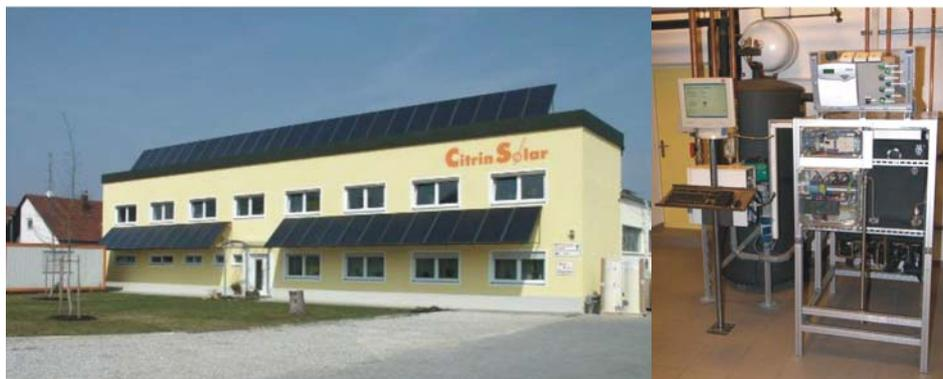
Figure 1: Solar air-conditioning system of CitrinSolar with flat plate collectors on the façade and on the flat roof as well as the chillii<sup>®</sup> STC6 adsorption chiller (sources: CitrinSolar)
