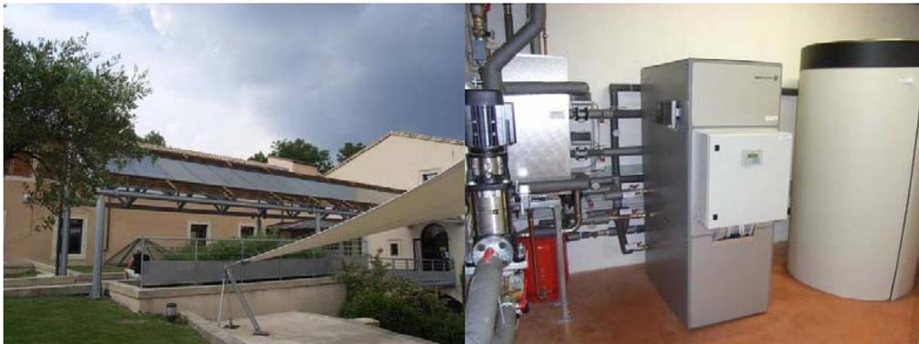
Figure 3: Building integrated flat plate collectors of the Haribo Museum in Uzés, France and suninverse 10 in the technical room (sources: Sonnenklima)
