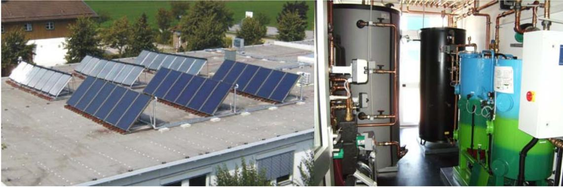
Figure 5: Flat plate and vacuum tube collectors on the roof of the SolarNext provide the chillii® solar cooling and heating system, the heart of the system is an EAW Wegracal SE15 (sources: SolarNext)
