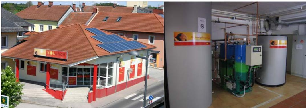
Figure 6: Flat plate collectors on the roof and EAW Wegracal SE 15 absorption chiller in the technical room of Sol-ution in Sattledt, Austria (source Sol-ution, EAW)
